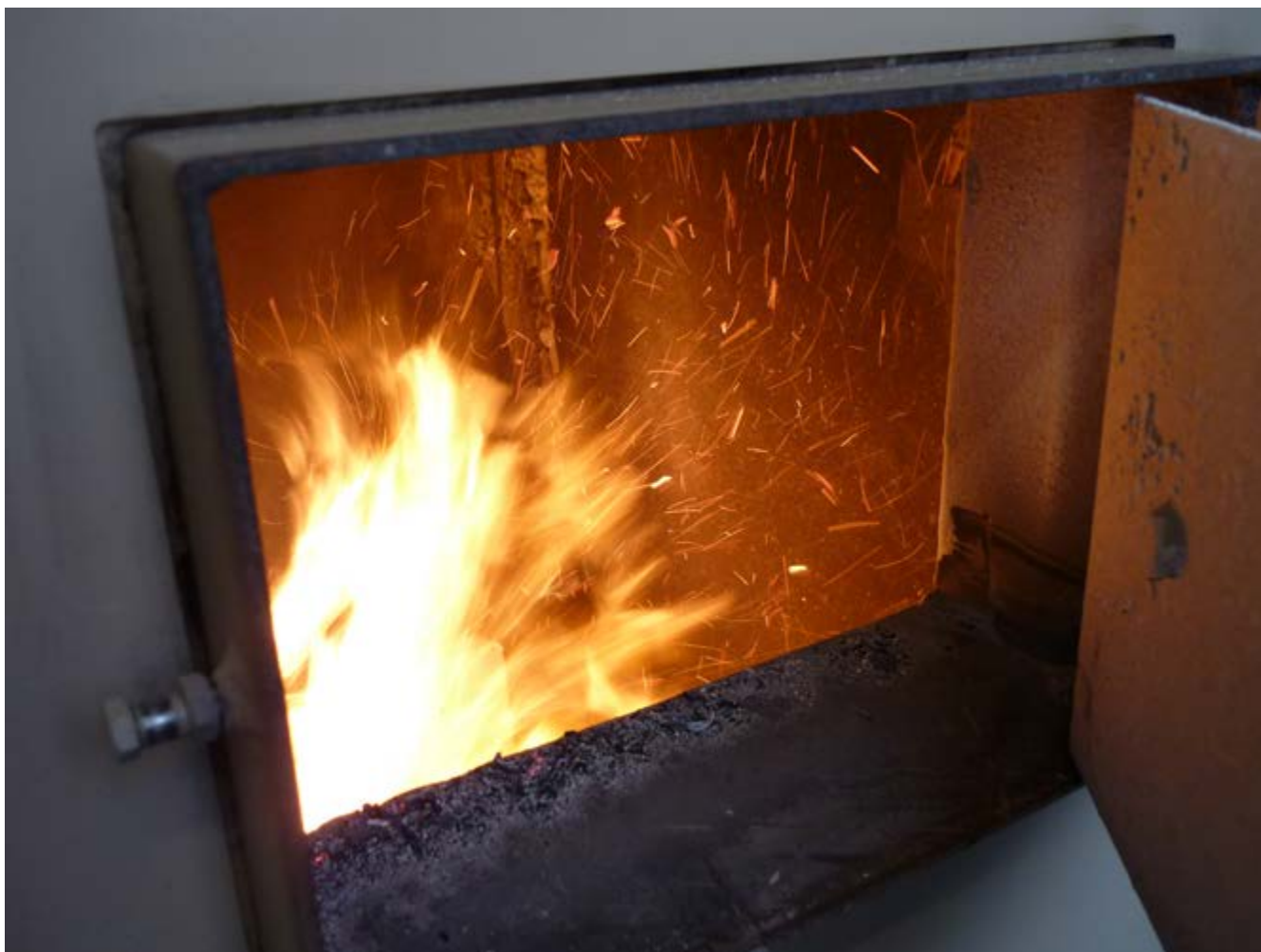
Combustion of willow, Veto boiler
